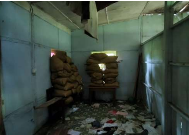
Construction of bunkers by terrorist insurgents inside the township public hospital in Thantlang town.
