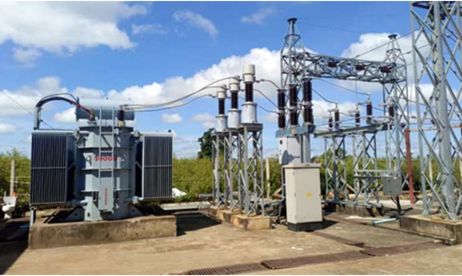
Photo record of the completed repairs of damaged substation equipment at the 33/11 kV 10 MVA Shwe Nyaung Pin substation in Nawngkhio Township.
