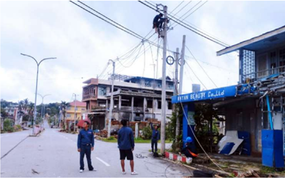
Photo record of electrical staff repairing the damaged 400V power lines.
