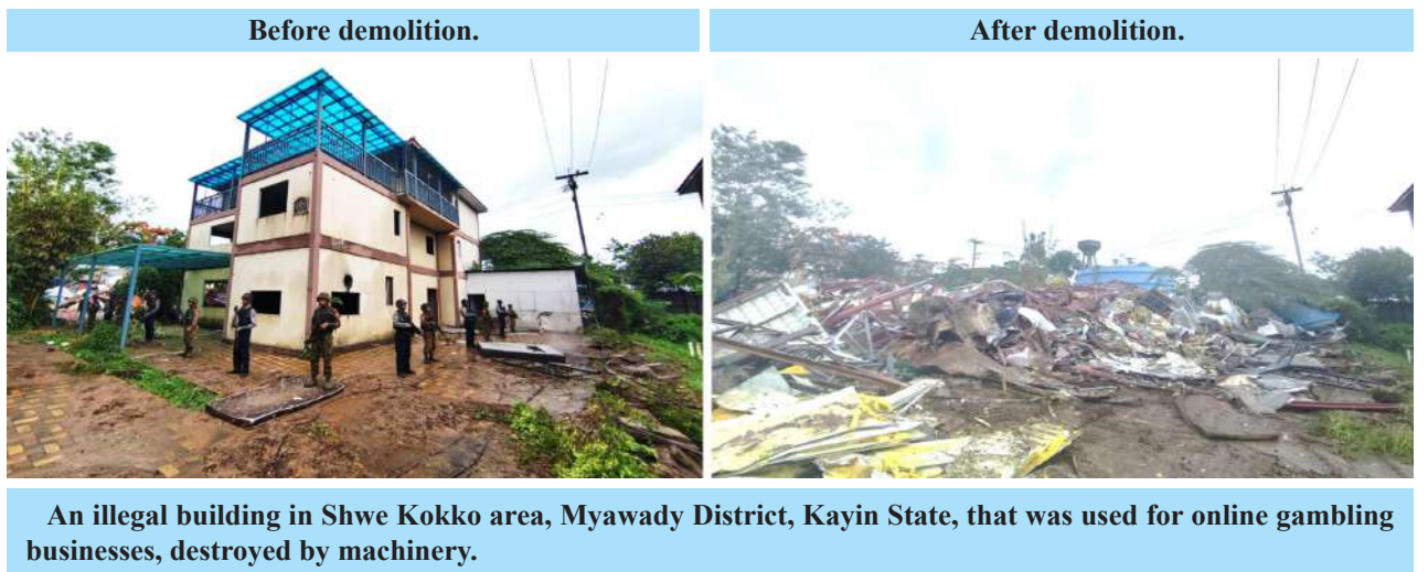
Destruction of illegal buildings used for online gambling businesses in Shwe Kokko area, Myawaddy District, Kayin State, destroyed by machinery.
