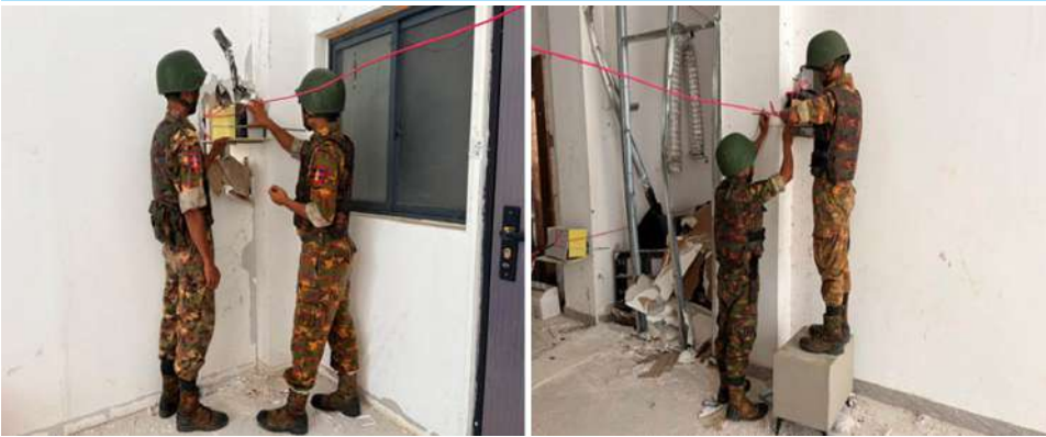
Preparation and placement of explosives.
