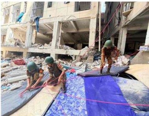
Rigging detonation cords for controlled demolition.
