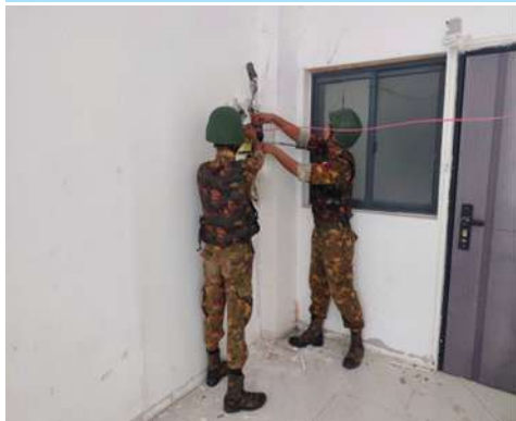
Preparing and setting explosive charges.
