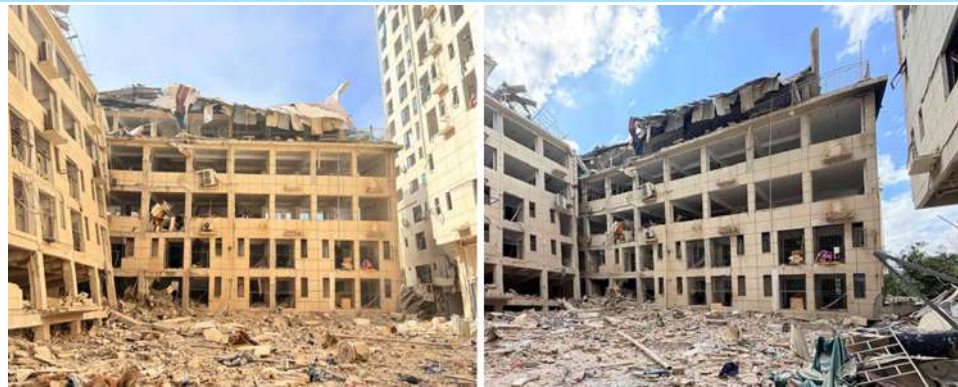
View after demolition.
